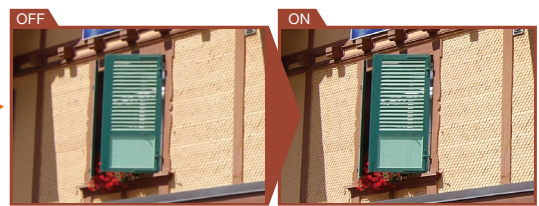
Increasing the resolution clarifies the unevenness of the wall, revealing a feeling of solidity and depth.
